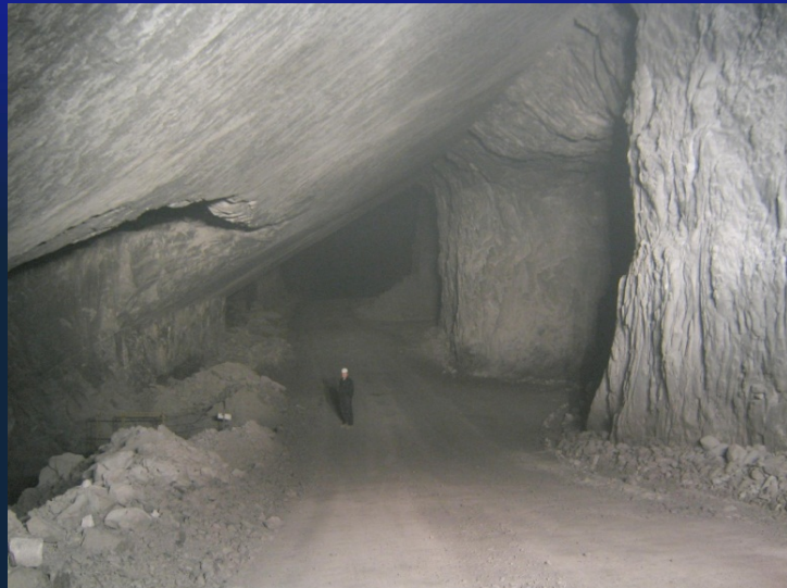
looking down 14 East #2 (top of escape-way ladder from 15 th level seen on left)
